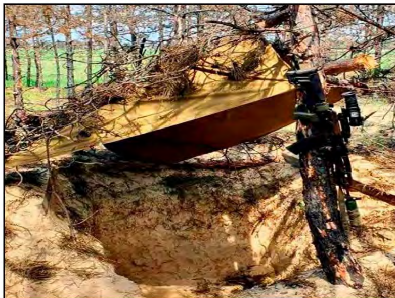
Fig. 6. Individual trench with a cover on top, camouflaged with pine branches from the surrounding forest.
